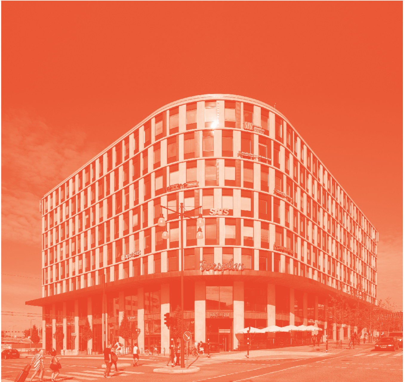
The SIS head office at Torsplan in Haga City in Stockholm, in one of Europe's environmentally top-rated office properties.
